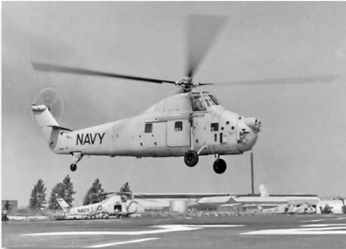
Sikorsky and the Navy tested the HSS-1F with T58 turboshaft power in 1957.
