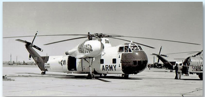
The Army CH-37B (S-56) ultimately snagged 2,500 lb loads in mid-air retrieval tests at White Sands Missile Range in 1962 and 1963. (Sikorsky Archives)
