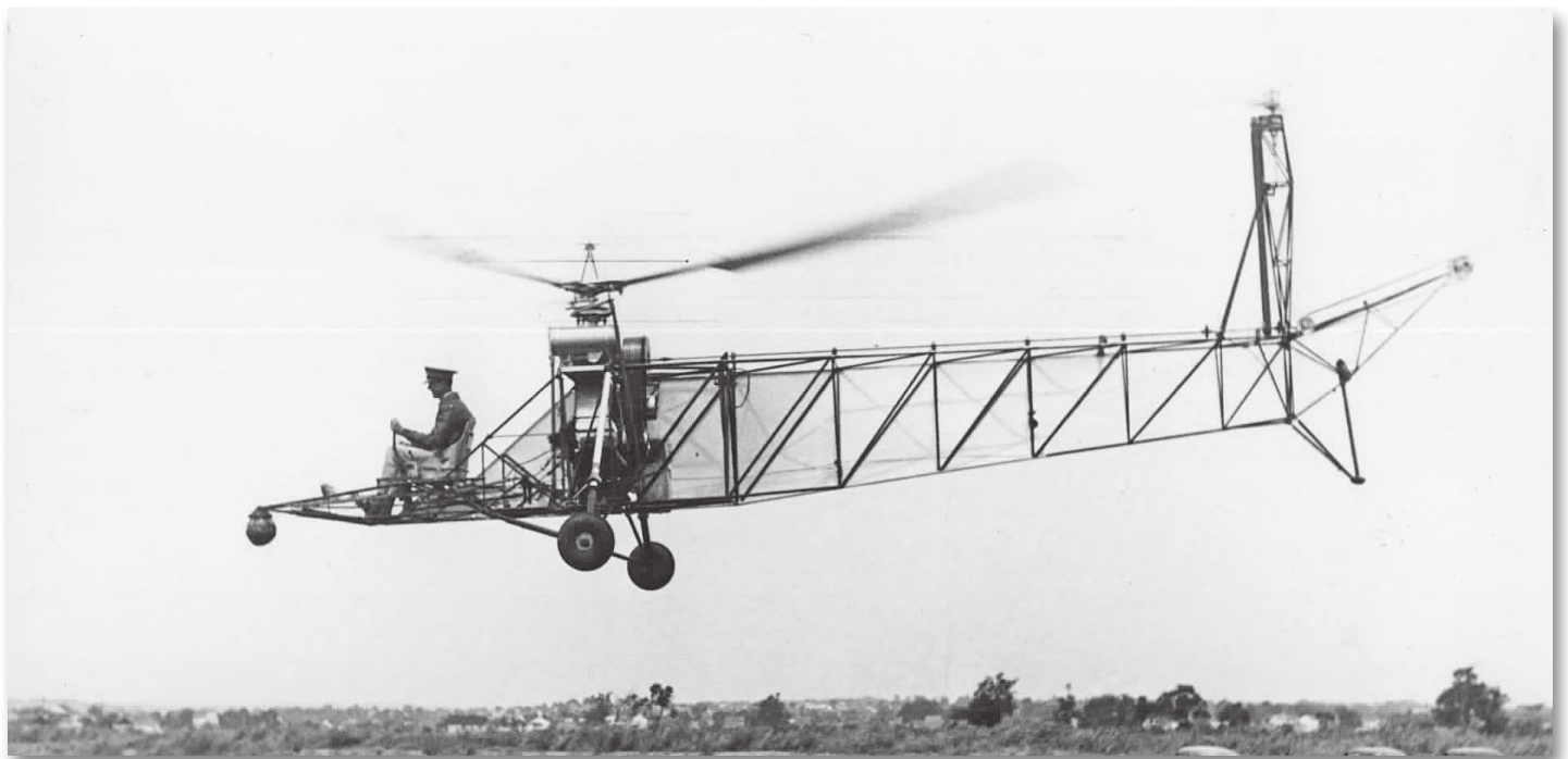
Throughout its career the VS-300 had only rudimentary cockpit instrumentation.
