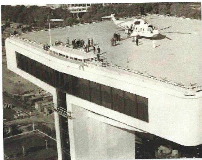
S-61 on New York Port Authority building roof
