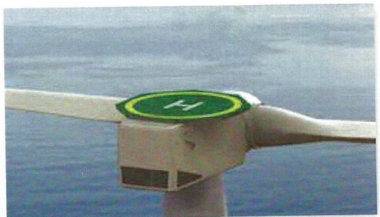
Helipad that is built on top of an air turbine structure
