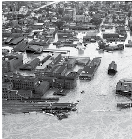
Waterbury, Connecticut Flood
