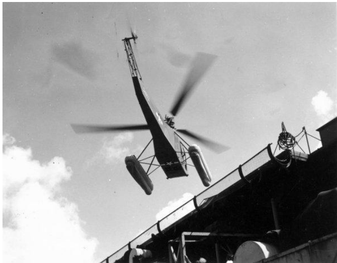
Figure 33: An R-4B wearing pontoons lands on the flight deck of one of the reconfigured Liberty Ships. The flight deck is over the forward cargo hatch at the front of the ship.
